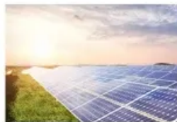
Energy Storage System
