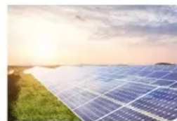
Energy Storage System
