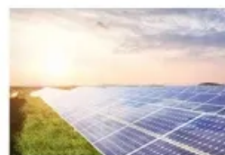
Energy Storage System
